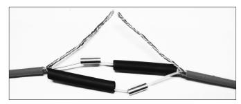
Centre 6" shrink tubing over exposed heating conductors. Shrink completely. Stop heating when excess sealant protrudes from both ends.
