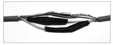
Allow the finished splice to cool down for 5-10 minutes. Measure insulation, total resistance and continuity.
