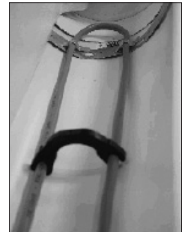
TXLP Cable with spacer and clip strip
