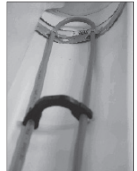
TXLP Cable with spacer and clip strip
